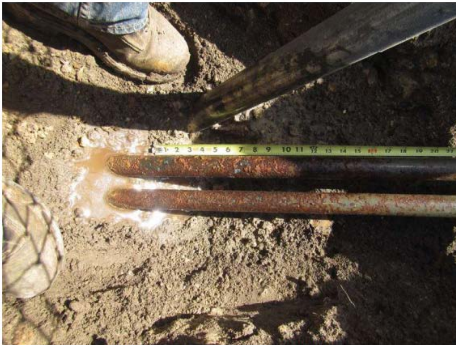
Photo 04_North Anchor - Anchor Shaft Below Grade
